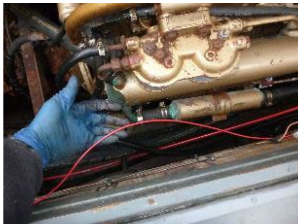
The positive wire for the fuel tank sender is not properly secured.
