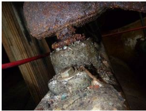
Starboard aft engine mount deteriorated.
