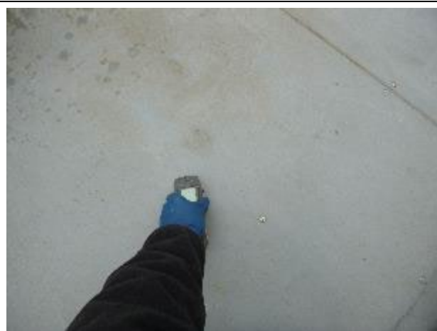
Elevated moisture in the removable cockpit sole panel to starboard. Meter reading 210.
