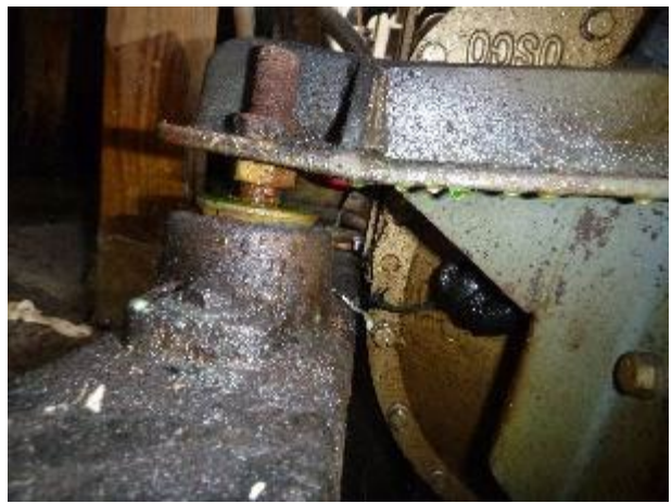
Antifreeze dripping of the port aft engine mount from a turbo leak.
