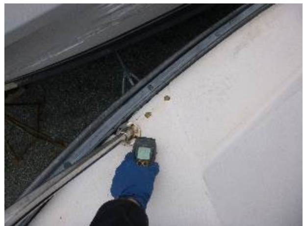
Elevated moisture in the foredeck. Meter reading 298.
