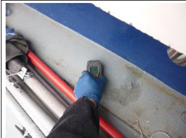
Elevated moisture in the cockpit sole to port. Meter reading 212.
