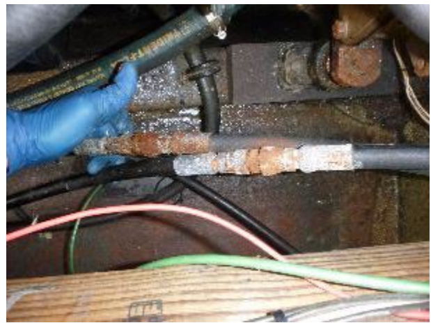
Steering hose connections rusted to starboard of the engine.
