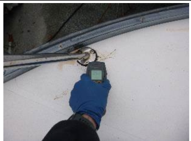
Elevated moisture in the foredeck. Meter reading 258.
