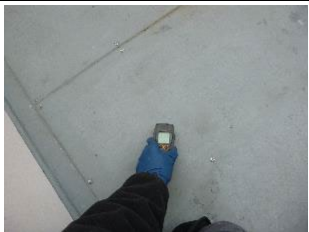
Elevated moisture in the cockpit sole to port. Meter reading 217.
