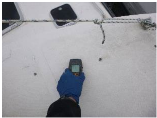
Elevated moisture in the hardtop. Meter reading 207.
