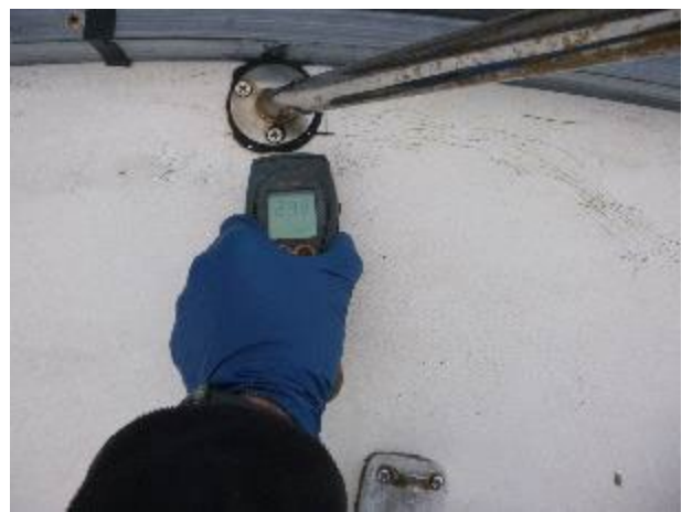
Elevated moisture in the foredeck. Meter reading 248.
