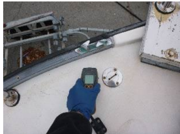
Elevated moisture in the foredeck. Meter reading 207.
