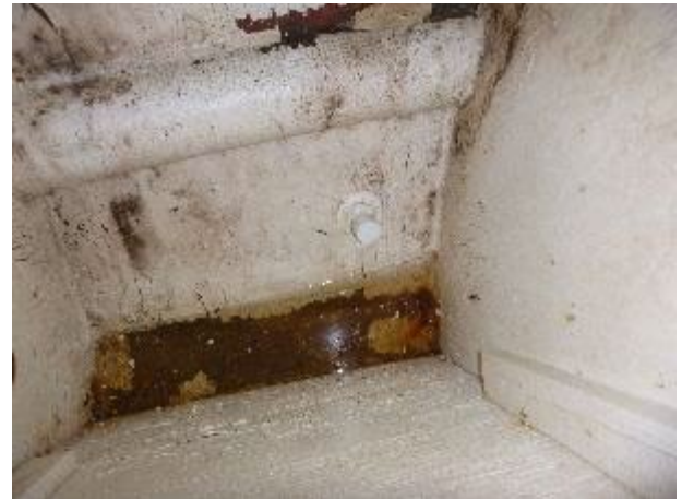
Standing water in several of the forward cabin stowages.
