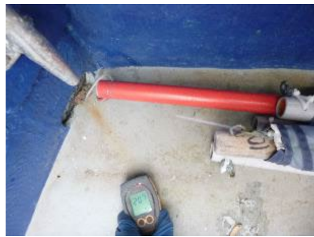
Elevated moisture in the cockpit sole aft to port. Meter reading 207.
