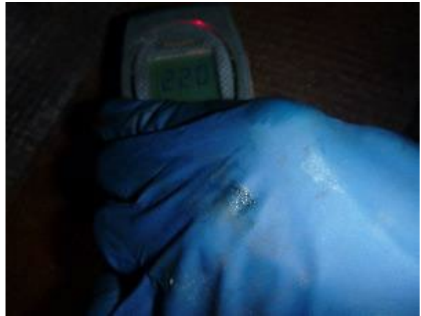
Elevated moisture in the starboard engine bed. Meter reading 220.
