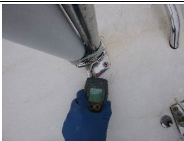
Elevated moisture in the hardtop, starboard forward. Meter reading 258.
