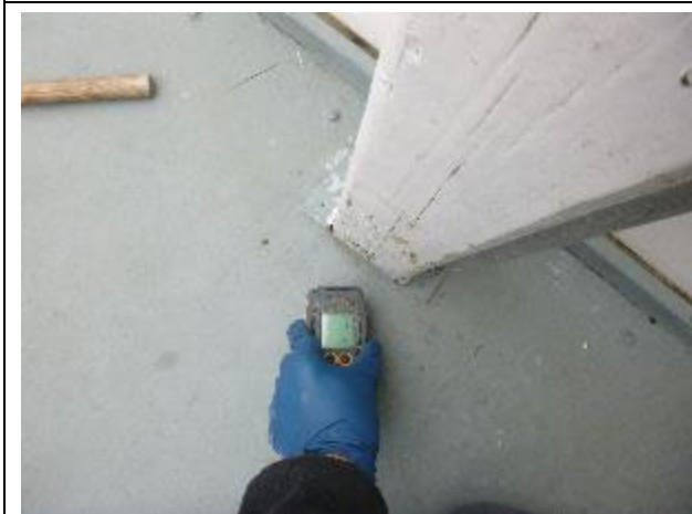
Elevated moisture in the cabinsole, forward to starboard. Meter reading 217.
