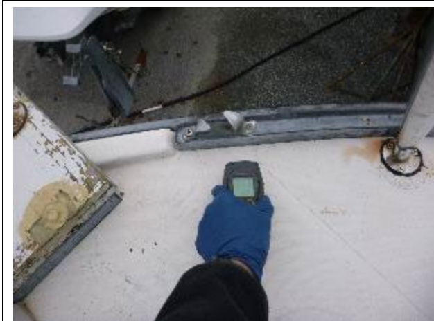
Elevated moisture in the foredeck. Meter reading 239.
