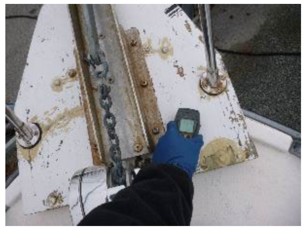
Maximum elevated moisture in the anchor pulpit. Meter reading 999.
