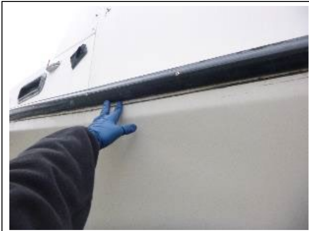
Port rubrail damaged and shifted.
