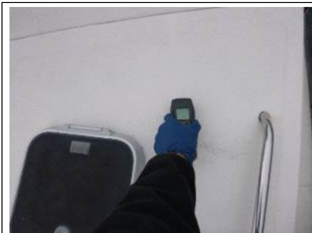
Elevated moisture in the port side top of the forward trunk cabin. Meter reading 215.
