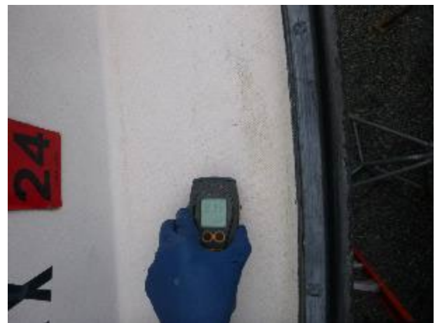
Elevated moisture in the starboard side deck. Meter reading 215.
