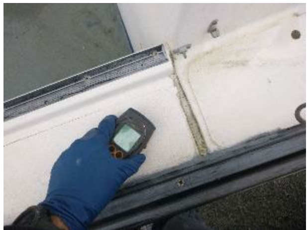
Elevated moisture in the starboard coaming top. Meter reading 287.
