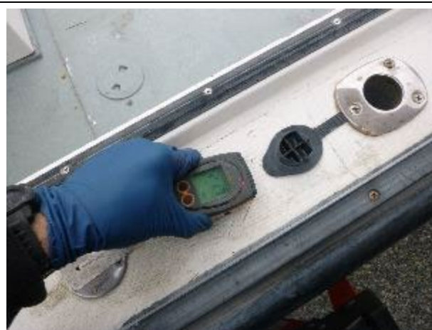
Elevated moisture in the port coaming top. Meter reading 217.
